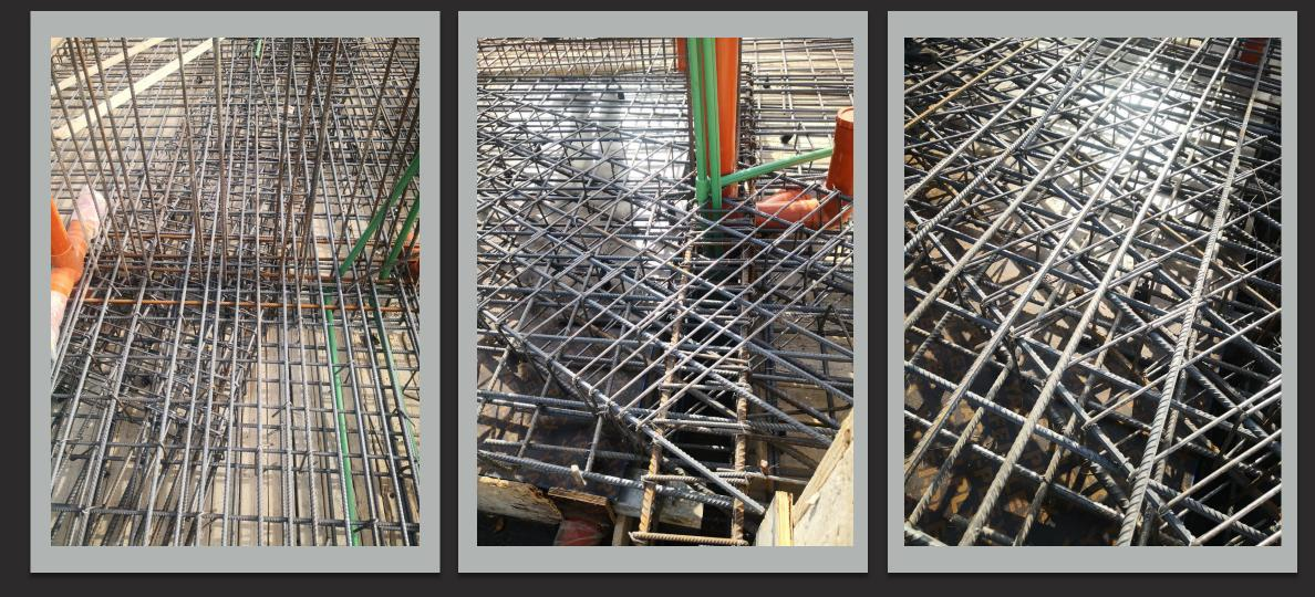
During the construction of this new kitchen space, steel rebars are carefully placed to structure the beam and columns, providing the essential foundation for stability. Meanwhile, mechanical installations are being integrated between the rebars, ensuring optimal performance and efficiency in the final design.
